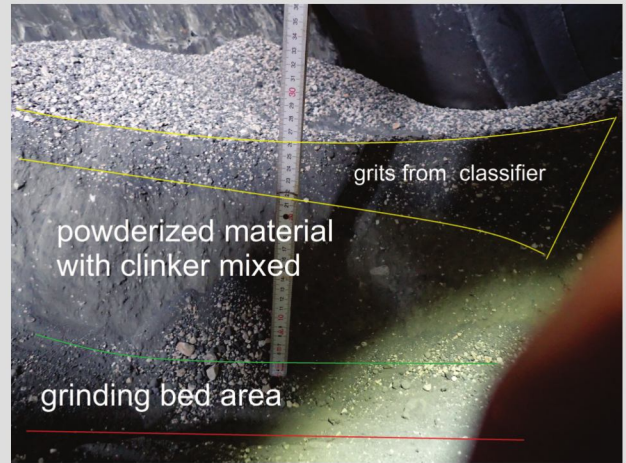
Picture 2: Profile of a grinding bed inside cement mill
